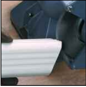
Removing burrs from the edge of a section of gutter with an abrasive nylon wheel brush.
