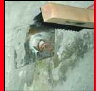
Removing excess concrete from the surface of a steel support plate.
