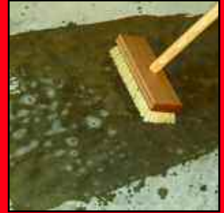
Scrubbing a concrete floor prior to painting.
