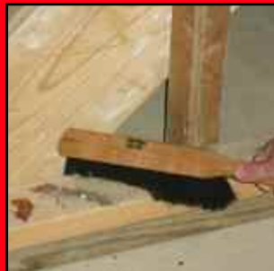
Sweeping dirt and debris from between studs.
