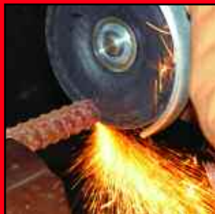
Cutting a piece of rebar to length.
