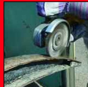
Prepping a machine guard for on-site welding and repair.
